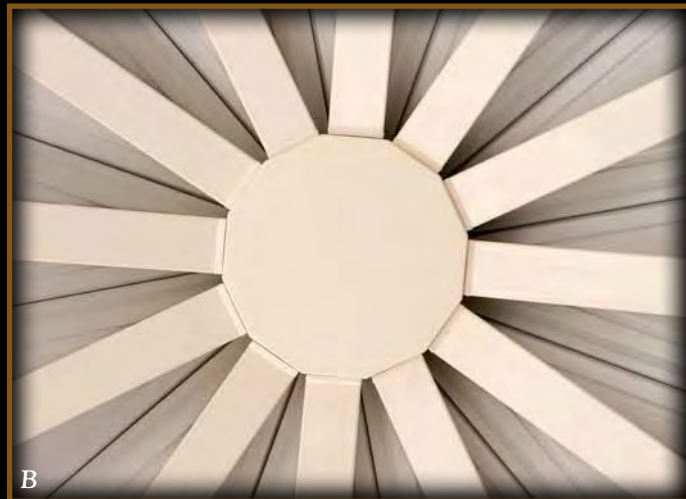
Detail of 60' model center compression ring, showing twelve beam connection.
