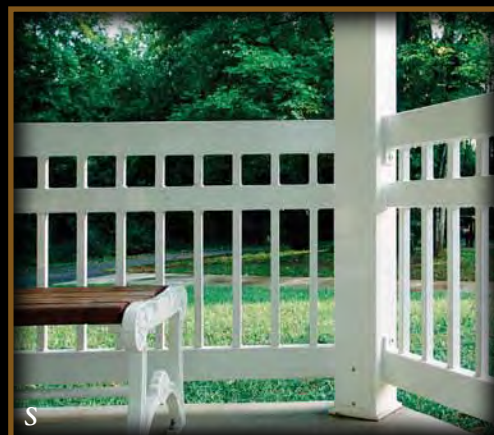
Heavy duty railing has 1" square pickets spaced 5" o.c. with tube steel rails
