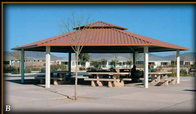
Sierra Verde, Glendale, AZ: With a second tier to facilitate airflow, this 36' model features a 4:12 pitch in Terra Cotta colored HR-36 steel roof.
